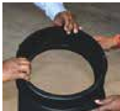
5 FIX RUBBER RING ON FRAME
