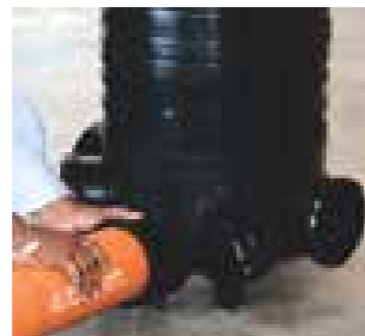
9 FIX FOAMCORE PIPE IN INLET
