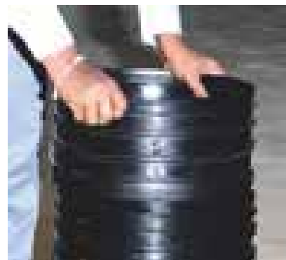
4 FIX ANOTHER RISER ON CHAMBER BASE
