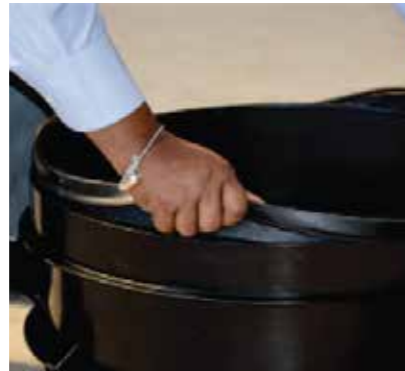
2 FIX RUBBER RING ON RISER
