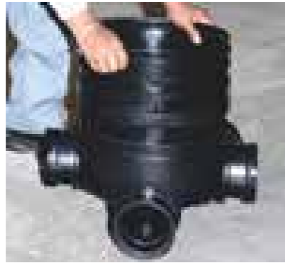
2 FIX RISER ON CHAMBER BASE
