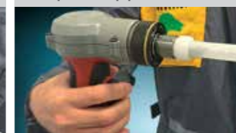
4. Insert the fitting in the pipe
