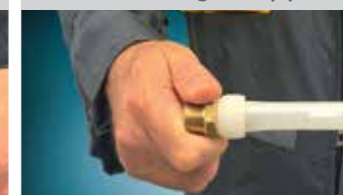
4. Insert the fitting in the pipe
